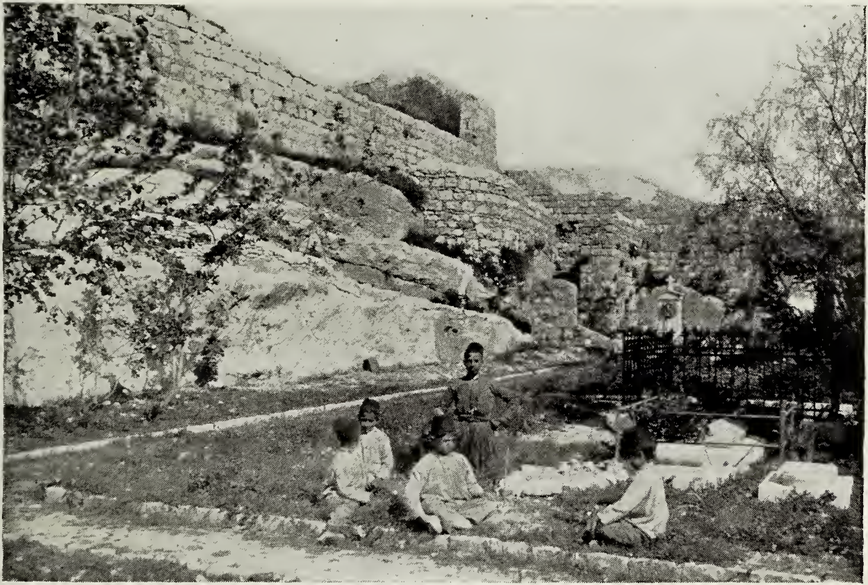
SITE OF OLD JEBUSITE WALL
